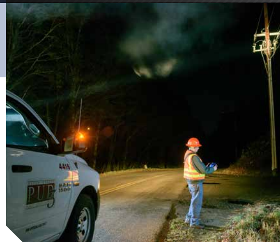
PUD 3 engineers perform the majority of their scans at night when the electrical load is greater.
