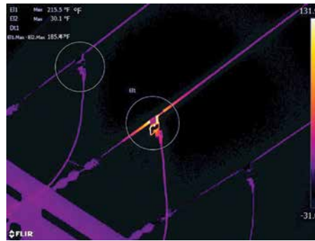
The center-phase hot tap is showing imminent failure. This hot line-clamp, or bail, connects two circuits together. A poor connection on the line clamp is causing heating on the primary line. Had it failed, 2,250 customers would have lost service.
