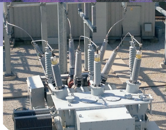
Typical equipment that is monitored by electric power utilities includes bushings, breakers, capacitor banks and high-voltage switchgear.
