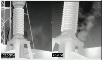
Optical gas imaging cameras visualize and pinpoint emissions so you don't have to shut down operations to fix a leak
