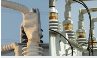
A bushing failure may cause extensive damage to a transformer and other equipment — and put personnel safety at risk
