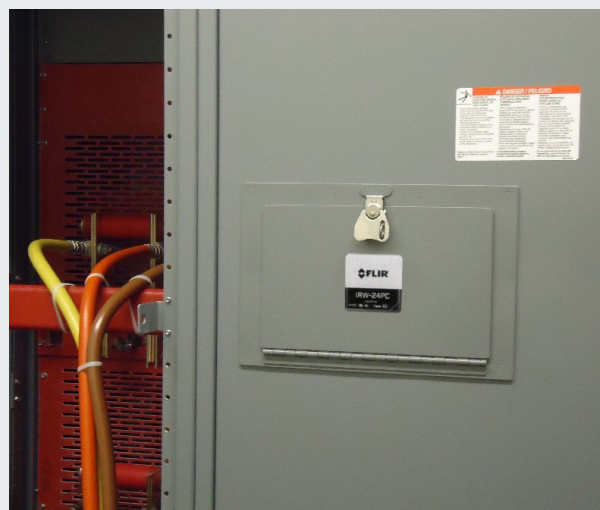
A FLIR IR Window creates a safe barrier between the inspector and energized equipment.
