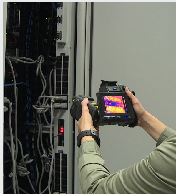
With a handheld thermal imaging camera, operations managers can find and diagnose problems, then verify the repairs.
