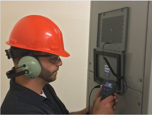
With a maintenance inspection window for visual, infrared, ultraviolet, and ultrasound inspections installed on medium voltage switchgear, no special PPE is required to use the EMSD
