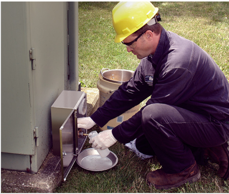
A safer oil sampling method retrofitted to an existing transformer allows energized sample collection; the sampling cabinet is lockable to prevent unauthorized access (Courtesy SDMyers)
