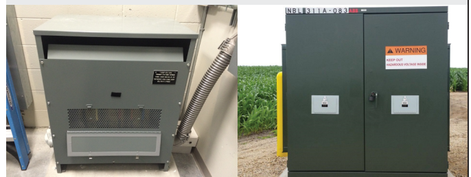
Custom replacement dry transformer panel-front with a built in maintenance inspection window
