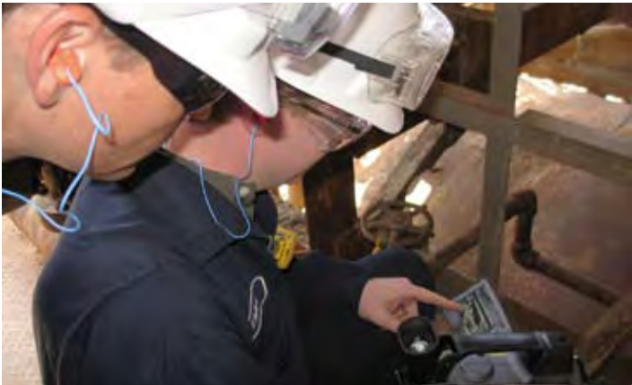
Co-workers the a location of a gas leak
