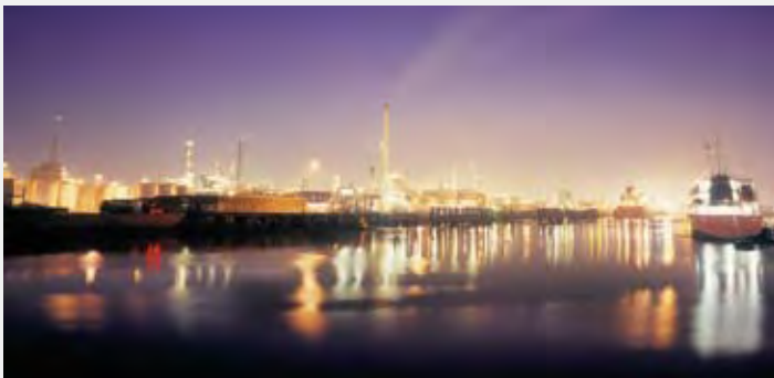
A modern complex petrochemical facility
